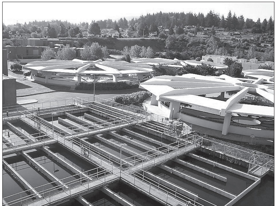
A portion of the sewage treatment plant at Post Point.
